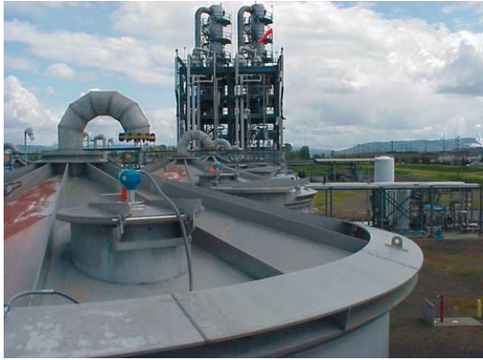
Micropilot M FMR240 installed in man hole covers of storage tanks.
