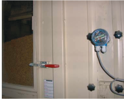
Mounting location of the Soliphant T
