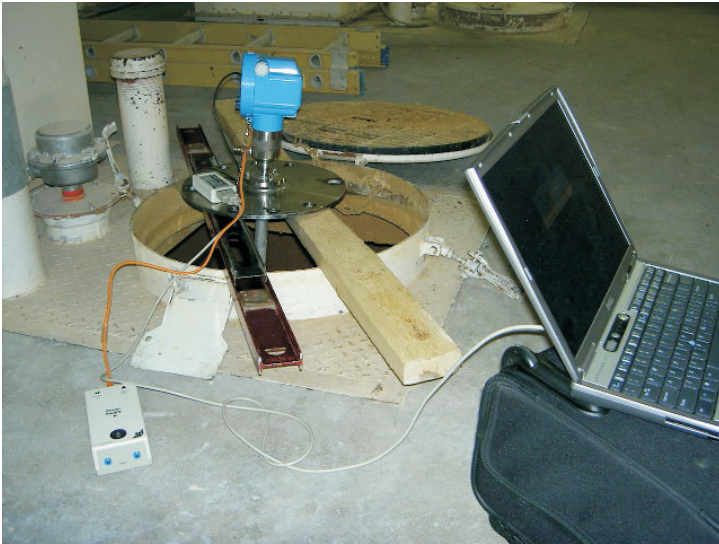
Simple set up and commissioning using lap top and ToF Tool
